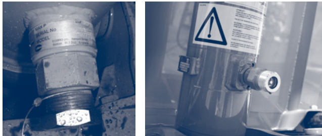
Figure 4.1.a. – Cylinder type plate + maximum cylinder pressure pictogram
