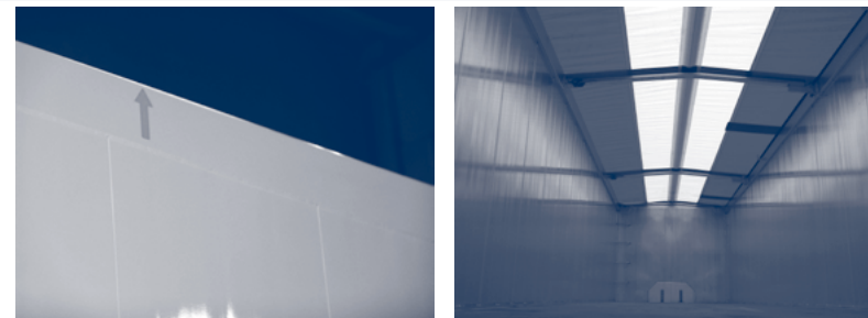
Figure 2.2.2.a. – Position of roof arches in the tipper (marked with red arrow)
